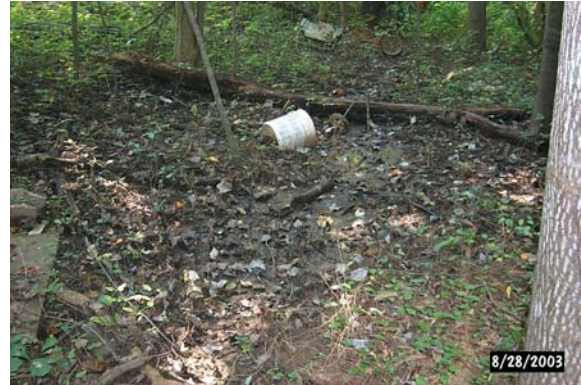
Fig. 6.4 Failed drainfield at Southwood MHP
