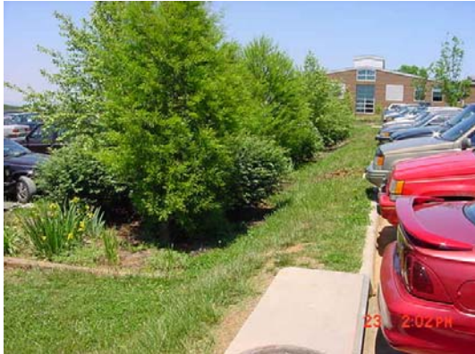
Fig. 6.3 Biofilter at Monticello High School, in the Moore's Creek watershed
