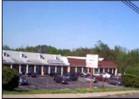
Potential station location at shopping center in Crozet (Albemarle County)
