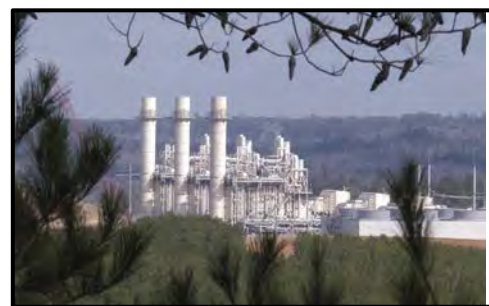
Figure NE-8, Tenaska
