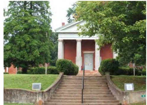
Figure LU-21, Historic Courthouse
