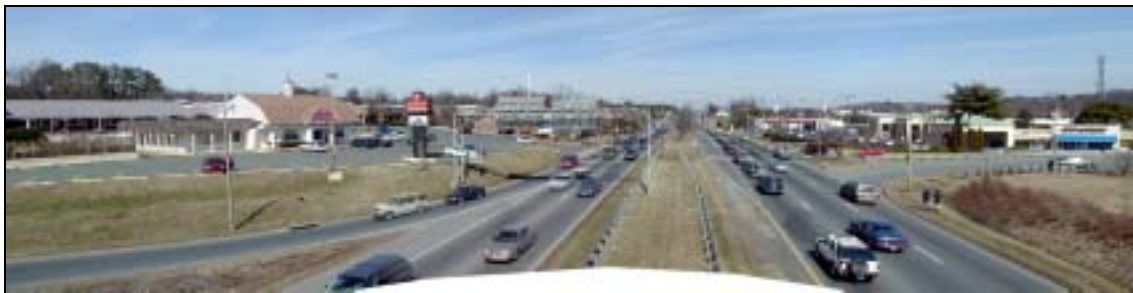
Figure 23 View from US 29/250 Bypass bridge looking north on US 29
