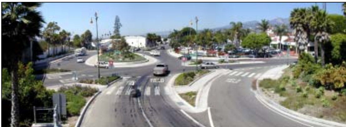
Figure 41 This Santa Barbara roundabout is at an off-ramp that meets a busy 5-way intersection and underpass
