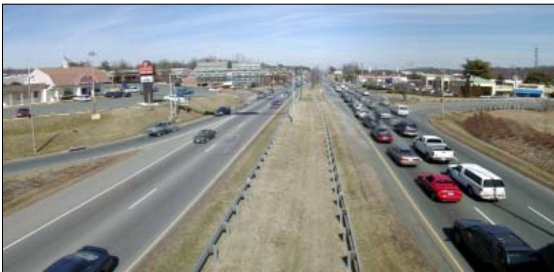
Figure 2 View From US 29/250 Bypass bridge looking north
