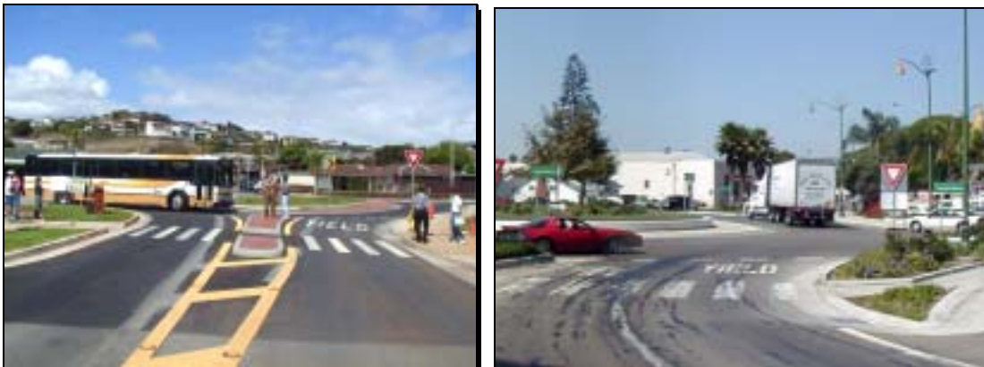
Figure 53 Well-designed roundabouts meet the needs of truck and bus traffic
