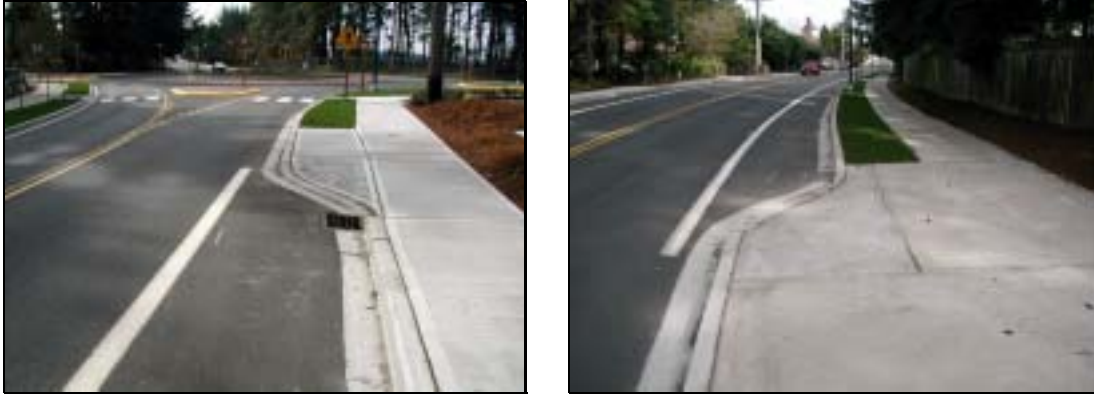
Figure 52 Bike lanes approaching roundabouts can have their own ramp onto the sidewalk, though most experienced riders will prefer to merge with the slow-moving traffic
