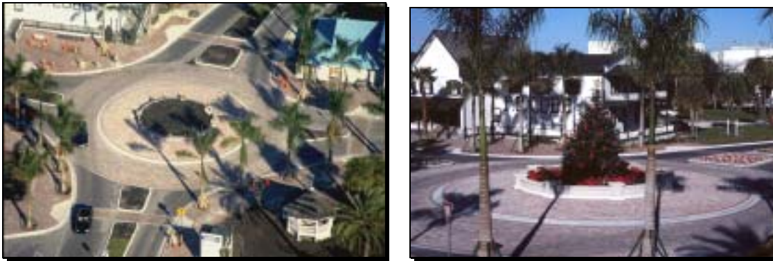
Figure 48 This Fort Pierce, FL roundabout replaced a signal at a four-lane state highway, creating a community focal point, while still moving traffic
