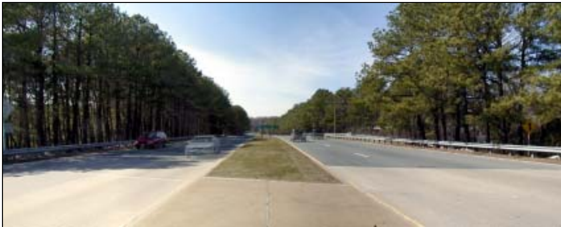
Figure 22 View of 250 Bypass over US 29
