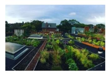
A green roof is a roof that is partially or completely covered with native vegetation, a growing medium, and a waterproof layer. Green roofs are designed to support plant growth and capture stormwater runoff.
