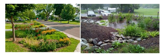
Bioretention cells and rain gardens are shallow depressions in the landscape planted with native plants and a specialized soil mix that can retain stormwater during rain events. These practices are designed to collect rainwater runoff from roofs, driveways, and sidewalks and allow it to slowly soak into the ground. Rain gardens allow at least 30% more water to infiltrate the ground than traditional lawns of the same size.
