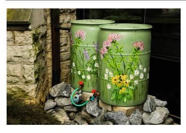
Rain barrels and cisterns capture rainwater from roofs and store it for later use, such as watering lawns and gardens, washing cars, or filling ponds. Collecting roof runoff in rain barrels reduces erosion near downspouts and the amount of runoff leaving a property. Rainwater is better for plants than municipal or well water, and it is a free water source for non-potable water use on your landscape. Rainwater harvesting is a simple and effective way to conserve water. Individuals can install
