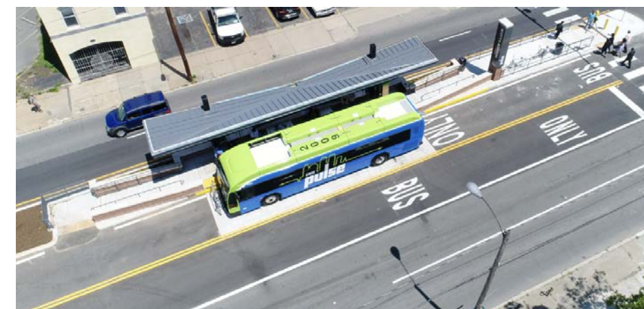
GRTC's Pulse line, showing some of the features of BRT like dedicated stops, dedicated lanes, distinct buses, and improved pedestrian access.
