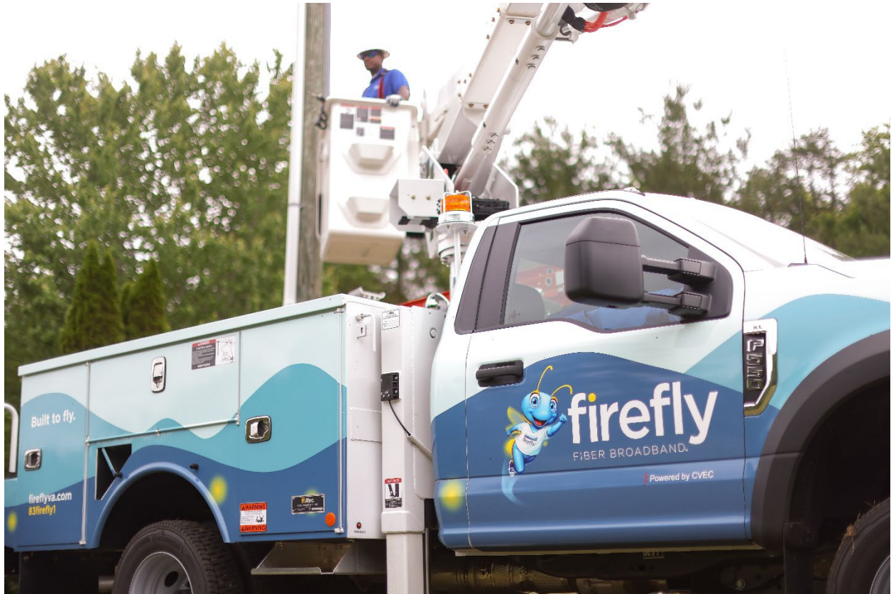
Firefly installer operates a bucket truck in rural Nelson County. Photo credit: Firefly Fiber Broadband SM
