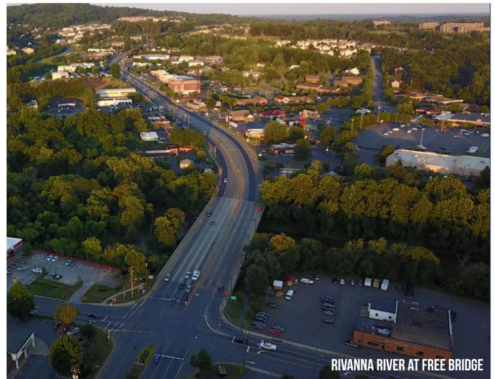
EXAMPLE OF BIKE & PEDESTRIAN BRIDGE IMAGE COURTESY OF SMITH SECKMAN REID, INC.
