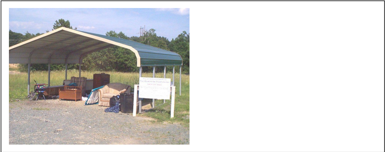
FIGURE 3. REUSE FACILITY IN FLUVANNA COUNTY
