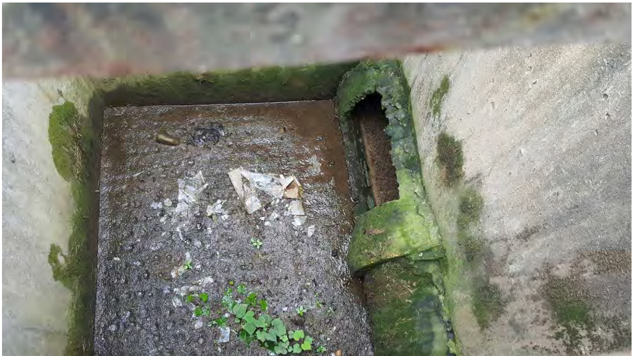
Image 2. Drainpipe within drainage inlet structure.
