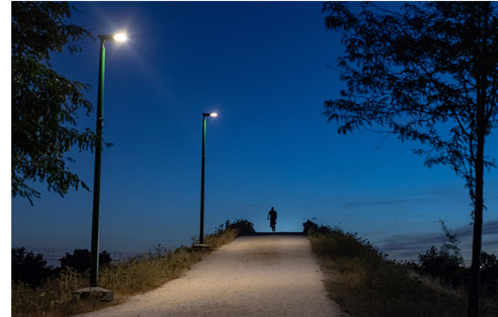
Example of trail lighting: Image courtesy of signify.com
