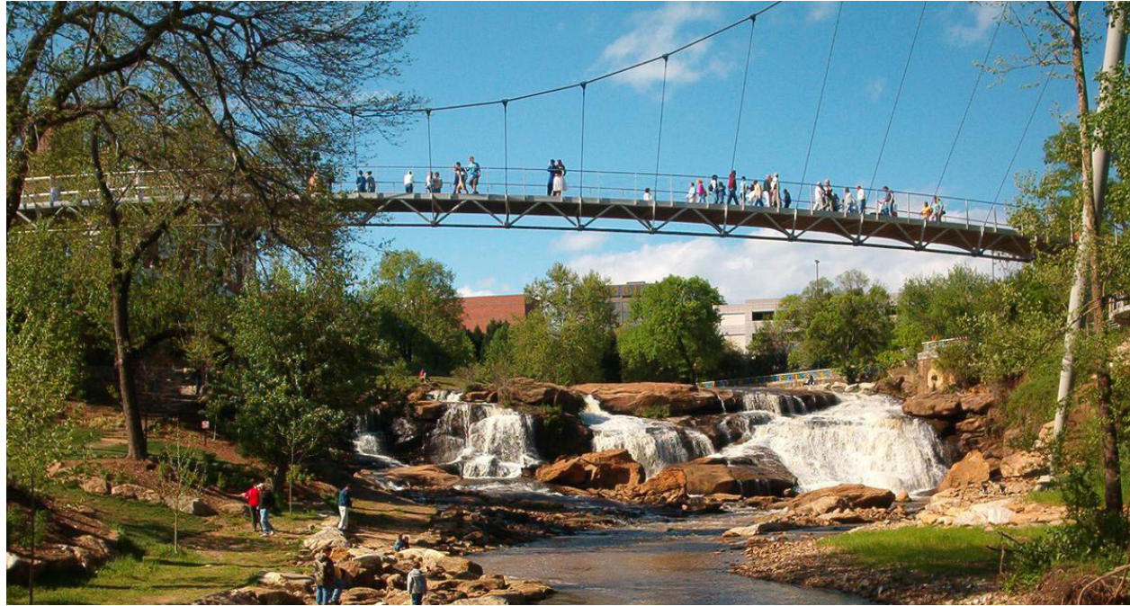
Liberty Bridge: Image courtesy of structurae.net
