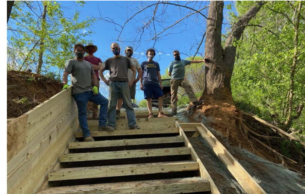
Volunteers build new access point along the Rivanna: Image Courtesy of Gabe Silver
